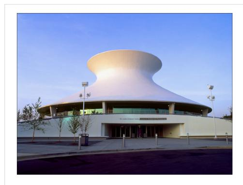
The St. Louis Science Centre Planetarium's exterior curved surface is in the shape of a **hyperboloid of revolution**. This shape is formed by revolving a **hyperbola** around its axis.
